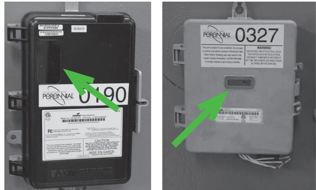
Load Control Unit Lights ~ irrigation well is controlled when both RED & GREEN lights are lit. When the GREEN light is the only light lit, the irrigation well is not under control.
