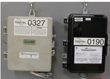
Left is the old style and the one on the right is the new load control switch.
