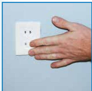
Install foam gaskets behind outlet and switch plates to prevent air leaks.
