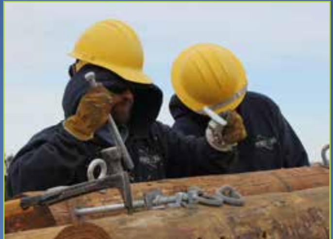
Shayde Linabery and Christopher Stutzman frame a pole.
