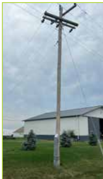
Reinforced Pole Using Galvanized Steel Support
