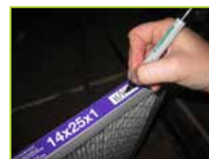
Mark when filters are replaced to keep them up to date. NRECA photo.
