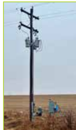
Irrigation well bank
