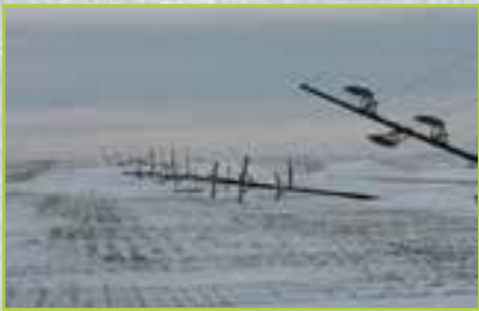
Damaged Sub-T line from the March 19th blizzard. Photo credit Rick Gerken
